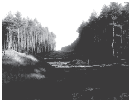
Fig. 2. Construction of the motorway around Olkusz (Poland) Interference with the natural environment (deforestation) (Photo by M. Gomułka)
