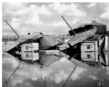
Fig. 1. Destruction of gas tank due to floods in Ostrava in 1997 [1]
