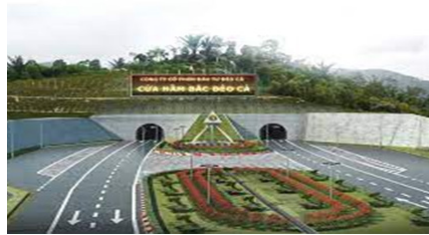
Fig. 2. Deo Ca traffic tunnel
